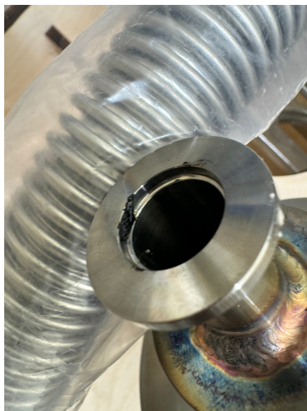
Figure 27 — Corrugated line connected to a nozzle. Corrugations, restrictions and transitions must be considered when assessing measurement-path conductance.
